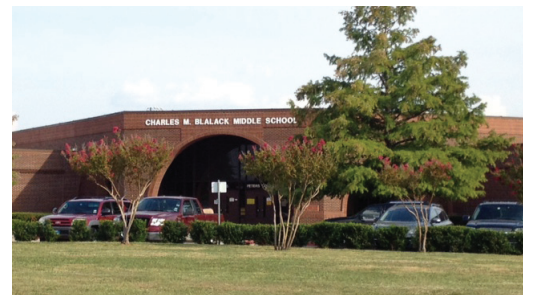
Blalack Middle School improves energy efficiencies by 20%.
